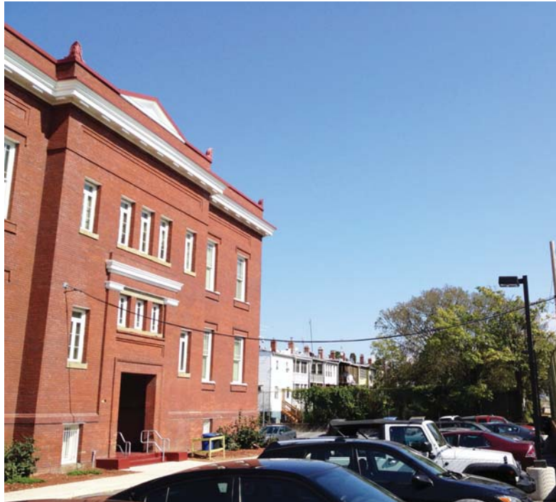
View 5 - Rear Alley / Parking Lot Looking East
