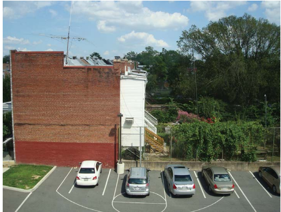
View 6 - Adjacent Rowhouse Facade
