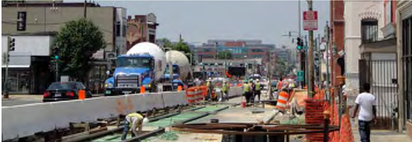
Construction of the H Street/ Benning Road NE streetcar segment, August 2010
