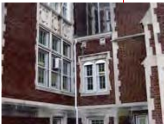
EXISTING SECURITY GRILLE Replace existing metal grille and windows with new security glazing at lower two floors, per DCPS guidelines, typical throughout.
