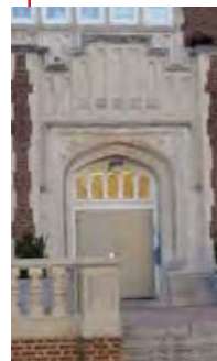
EXISTING EXTERIOR DOORS Replace existing metal doors with new paneled doors per DCPS guidelines and historic photographs, typical throughout.
