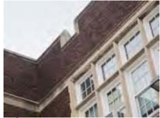
EXISTING STONE Clean existing stone and repoint as necessary - typical throughout
