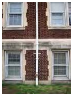
ROOF DRAINAGE Replace existing downspouts with new metal downspouts to match existing metal flashing - typical throughout
