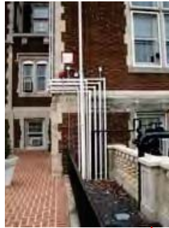
MEP ELEMENTS Existing piping and conduit to be removed and concealed within the building - typical throughout
