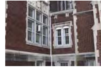
EXISTING SECURITY GRILLE Replace existing metal grille and windows with new security glazing at lower two floors, per DCPS guidelines, typical throughout
