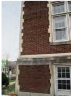
EXISTING STONE Clean existing stone and repoint as necessary - typical throughout
