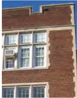
EXISTING WINDOWS Replace existing windows with new low-E windows per DCPS guidelines, typical throughout.
